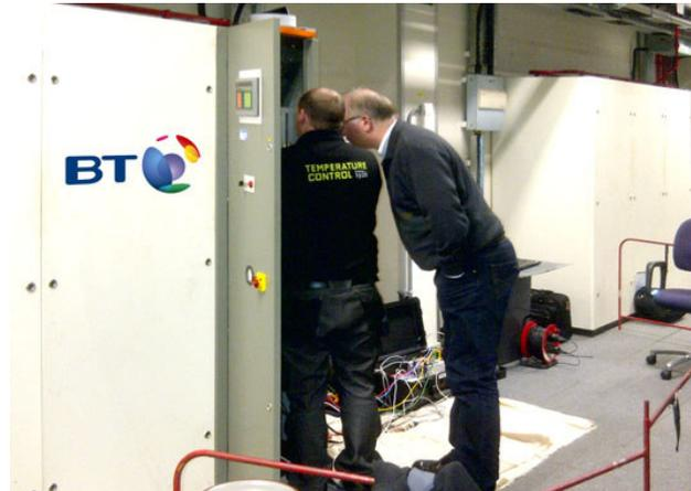
*Temperature Control managed the conversion of the 17-year-old GEA Denco close control system to ISCEON® MO99 at the British Telecom data centre in West London. The DuPont refrigerant closely matches the characteristics of R-22 for a quick and seamless replacement.*
