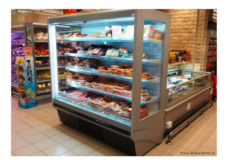
Following the launch of Opteon™ XP40 (R-449A) by Chemours in 2014 and the subsequent approval of this refrigerant by a number of compressor and cabinet manufacturers as an alternative to R-404A, Lowe decided to offer this as an option to their customers.Opteon™ XP40 has a GWP below 1400 and very similar performance to R-404A in retrofit and new equipment.
