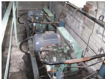
Fig. 1 Bitzer open drive reciprocating compressors
