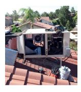
they have elastomeric seals. There's no need to replace Teflon® or nylon rings." After replacing the seals, he changed the filter dryer, evacuated the system to 500 microns, and charged the unit with ISCEON® MO99 refrigerant, with a weight just under the original system specifications. After allowing the system to stabilize, he added approximately 200g more of refrigerant.
