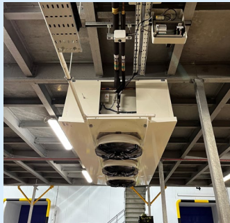
Dual Discharge Evaporator
