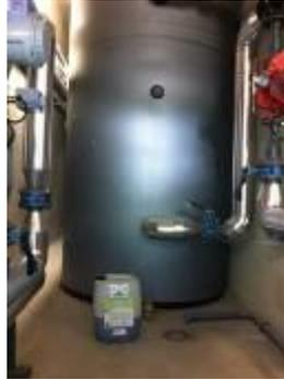
Because it has low expansion rates at high temperatures, it made it possible to size the expansion vessel accurately, thus reducing the overall cost of the installation. Alexandre Priquet (Bourrié) comments, "The fluid is very stable, and we have not seen any failure to increase pressure in the network. In addition to its technical characteristics, the fact that it is plant-based is also a plus for the whole system."
