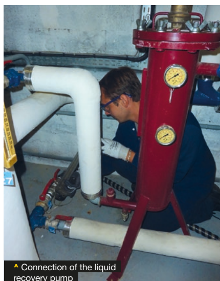
▲ Cleaning the magnetic filter (elimination of iron oxide)
