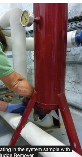
▲ Connection of the liquid recovery pump
